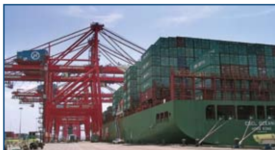
A pacific port cargo facility.
