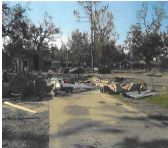
A foundation slab in the Gulf Coast Region
